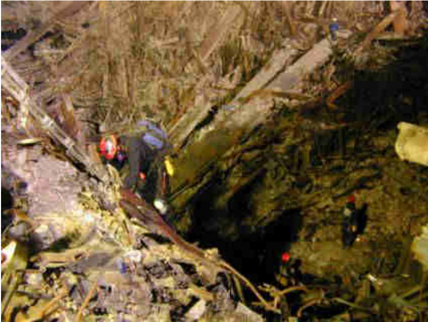
Figure 4-1 - GZ workers descend into the subbasements below WTC2. While there is extensive damage, there is little building debris at the bottom of the hole. There is no sign of molten metal. A worker in the distance walks along a massive core column. (photo filed 9/18/01) 86
