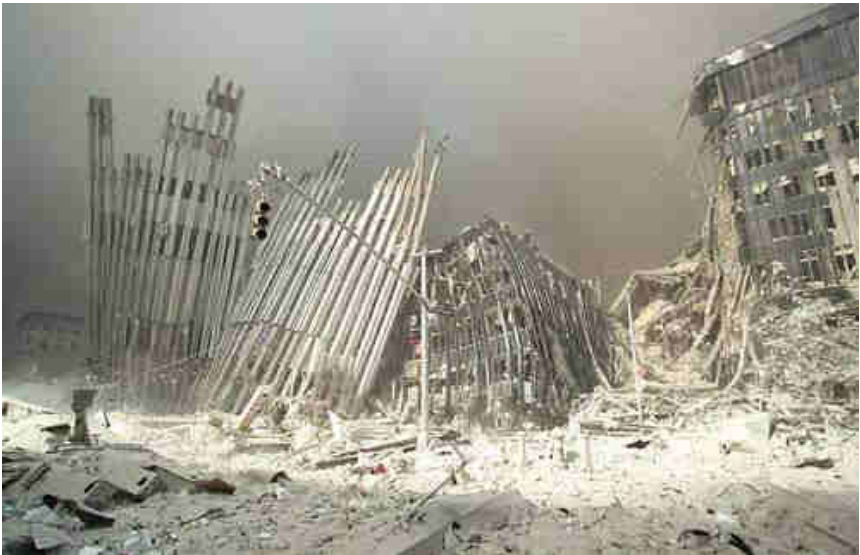
Figure 9-7 - The north wing of WTC4, as viewed from Church Street, looking west, appears surgically removed from the main body of WTC4, which has essentially disappeared. If WTC2 fell on it and squashed the main building, where is the part of WTC2 that did this?
